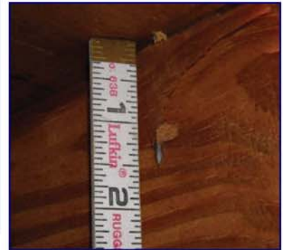
The inspector measures shiners to determine the nail size.
