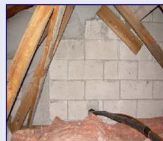
Reinforced masonry gable end.
