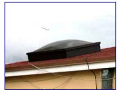
EVERY OPENING, including skylights and gable vents, must be protected in order to receive the Hurricane rating.
