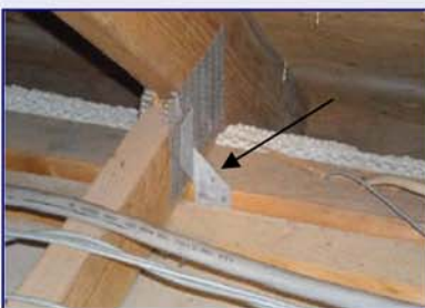
This photo shows clips as the roof to wall attachment.
