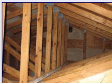
This is an example of 'Unbraced Gable End.'
