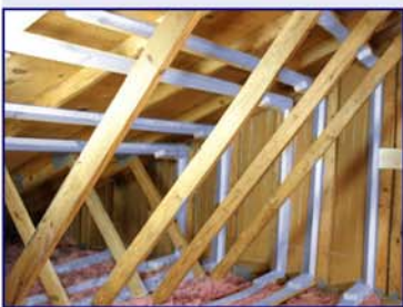
This photo shows one form of bracing called horizontal or continuous gable bracing (white boards).
