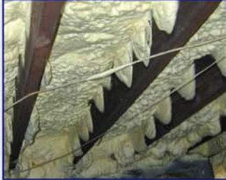
LEFT: A qualifying SWR for OIR 1802 purposes. Notice the seal is typically only along the joints.
