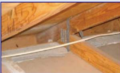
This photo shows a single wrap as the roof to wall connection.
