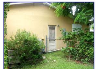
This home had every opening BUT this one protected. Because the glazing on this door is not protected with an impact resistant product, the ENTIRE home is classified as None.
