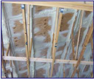
RIGHT: A photo of foam insulation, which does NOT qualify as an SWR.
